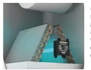
UVC-Advantage's small size allows for flexible mounting in the air conditioner. It will disinfect coil, drain pan, blower and other surfaces.
