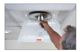
(SCVH VAV Heating) For a cooler room temperature, rotate red actuator clockwise. For a warmer room temperature rotate red actuator counter clockwise. Each full rotation will equal approximately + or  $-2^{\circ}$ .
