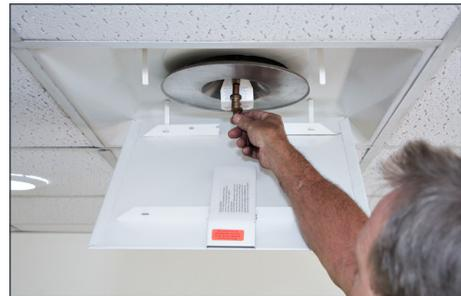
(SCVH VAV Heating) For a cooler room temperature, rotate red actuator clockwise. For a warmer room temperature rotate red actuator counter clockwise. Each full rotation will equal approximately + or - 2°.
